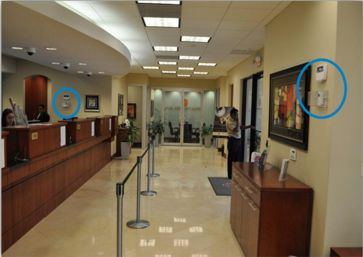
Two ECO3 units were mounted inside the bank, above the existing thermostats, so that savings could be easily checked by the staff.
