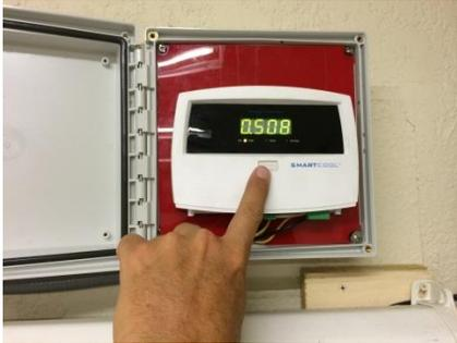
Note the yellow LED and the run data "0.508" which means 508 run hours accumulated (the "." point is actually a comma).
