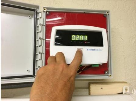
Note the RED LED is blinking and the override data of "0.283" which means 283 hours of compressor run time accumulated in override mode.
