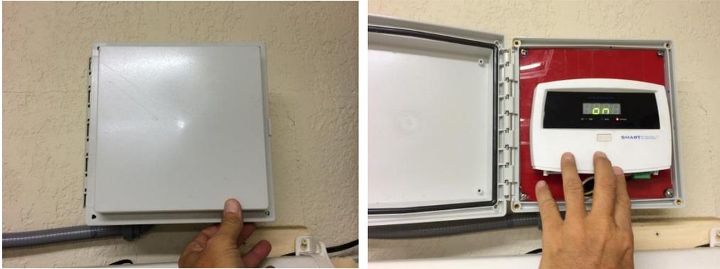
It might be outside next to the condensing unit in a box (usually with one screw to remove). Or it might be mounted on or near the air handler. Sometimes it is mounted on the wall next to the thermostat.
