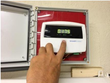
Note the green LED and the save data "0.175" which means 175 save hours accumulated.
