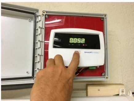
Note the RED LED is solid (non-blinking) and the bypass data of "0.052" which means 52 hours of compressor run time accumulated in bypass mode.
